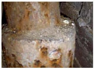
**Fig. 2:** The socket joint of an iron pipeline installed in the Octagon Source: H. Roscher – photographed on 11 March 2010
